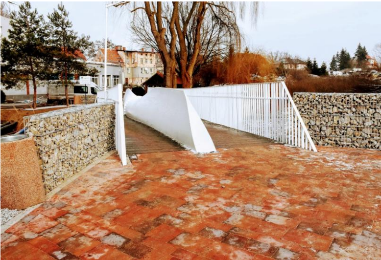
Bicycle and pedestrian bridge in Szprotawa, Poland (Source: GP Reblade)
