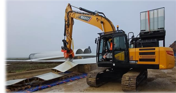
Circular saw cutting
