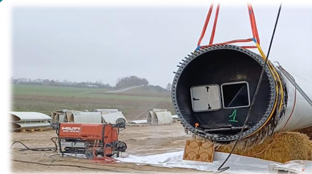
Wire saw cutting
