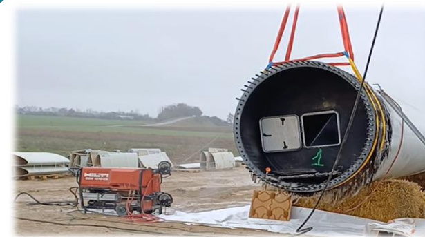
Wire saw cutting
