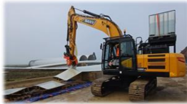
Circular Saw Cutting
