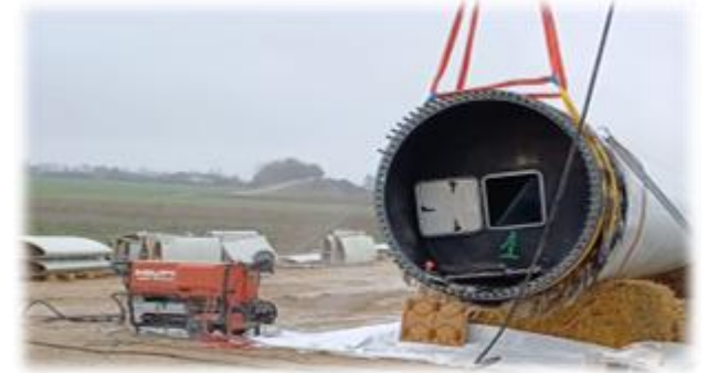
Wire Saw Cutting
